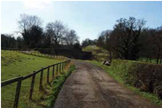
Bridge over the River Leven
